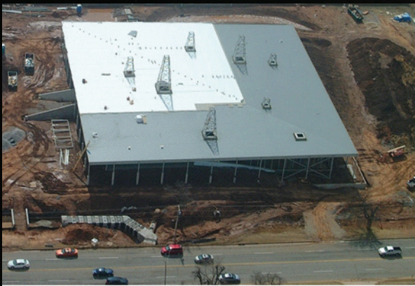
Aerial shot taken on Feb. 26, 2011
